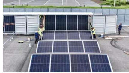
5G communication base station inverter under construction in
