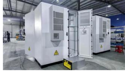
Warsaw battery station cabinet integration system
