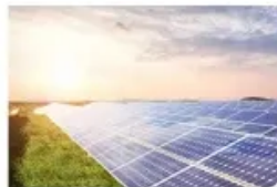
Energy Storage System
