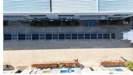
Tidal flat photovoltaic support structure
