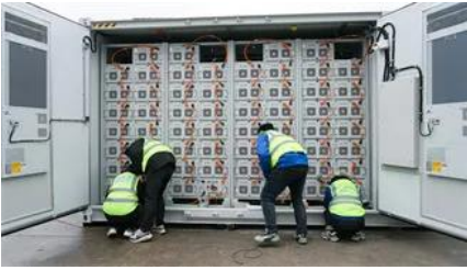
Communication base station inverter grid-connected lightning
