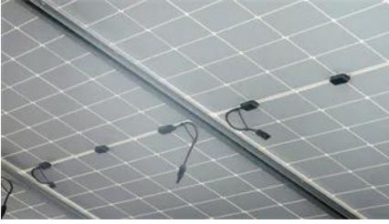
Supercapacitor solar power generation installation at Duodoma
