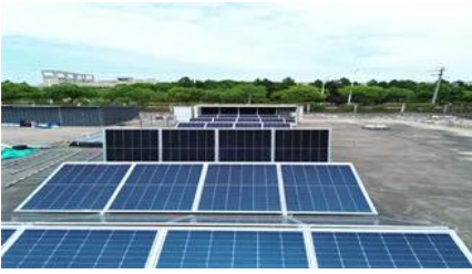
Micronesia 5g solar telecom integrated cabinet smart charging pile
