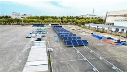
Envision Solar , Solar Panel Installation , Phoenix AZ
