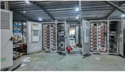
16kW Solar System w/ 30kWh Enphase Battery Backup
