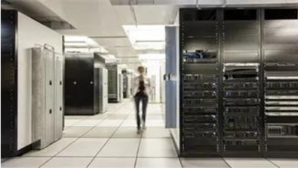
150kW Communication Power Supply Cabinet in Brazil
