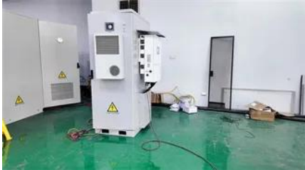
Port Vila Microgrid Energy Storage Battery Cabinet 20MWh
