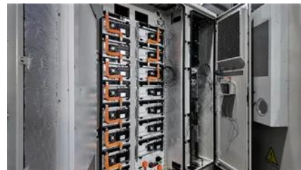
Port Vila Microgrid Energy Storage Battery Cabinet 20MWh
