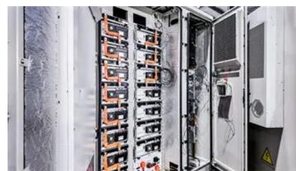
Outdoor Battery Storage Cabinet , TOPBAND LiFePO4 Energy
