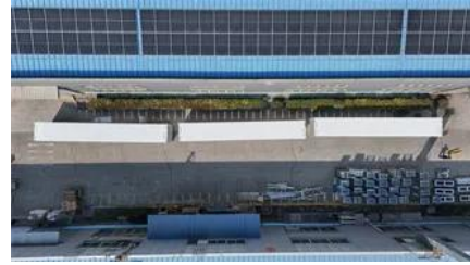
10kw Container Complete Set 3 Phase off Grid Solar
