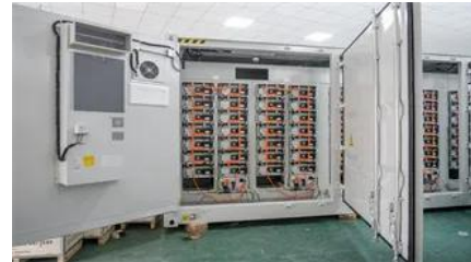
Niger outdoor telecom cabinet hybrid , ICEENG CABINET
