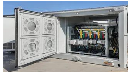
600kW Mobile Energy Storage Container Used at Naypyidaw
