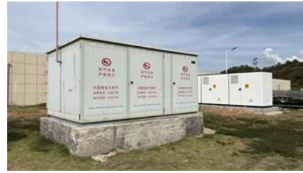
BMZ starts works on 65 mln euro battery plant in N.
