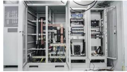
Jamaican photovoltaic container used at train station 40 feet
