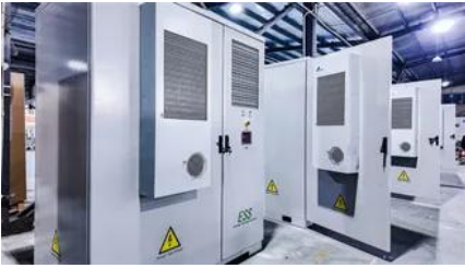
Deep Solar Ghana , Solar Installation in Ghana
