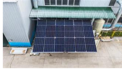
Large-Scale energy storage , Microgreen.ca
