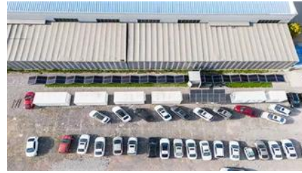
Guyana's Largest Hybrid Solar Plus Storage Facility Strengthens
