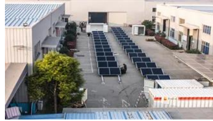
Lanshan County grid side energy storage power station starts
