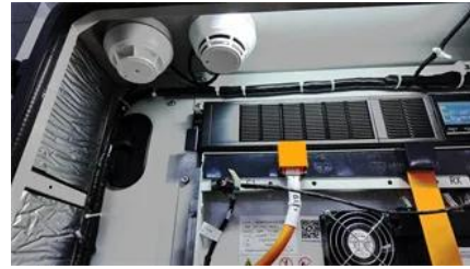
Building wind and solar complementary communication base
