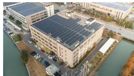
Energy storage container customization factory in the
