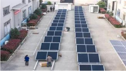
Cook Islands power grid energy storage power station construction
