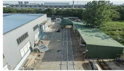
15 KV Siemens #GM-SG, switchgear with arc flash
