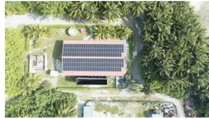
Cape Verde HJ Communication 5G solar container
