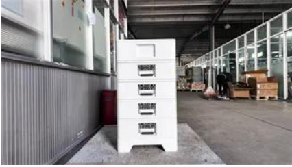
Botswana 5G communication base station flow battery construction
