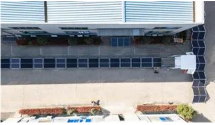
Skybox Pre-Wired Cabinets , Solar Batteries Online
