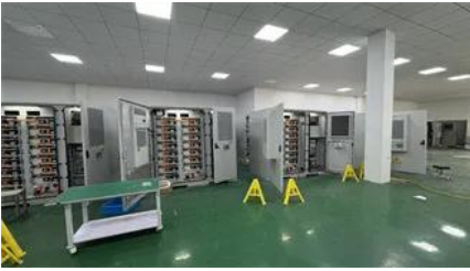
Munich Airport trialling new sustainable energy system
