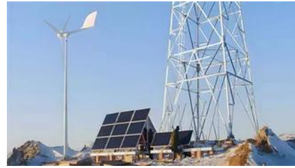
5MW Off-Grid Solar Container for Unmanned Aerial Vehicle Stations
