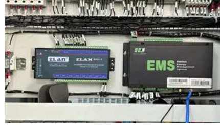
Bandar Seri Begawan wind power equipped with energy storage
